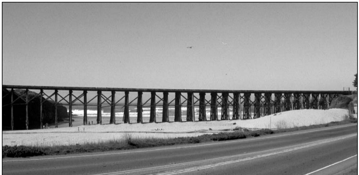
Trestle at Pudding Creek: A historically significant structure at MacKerricher State Park
