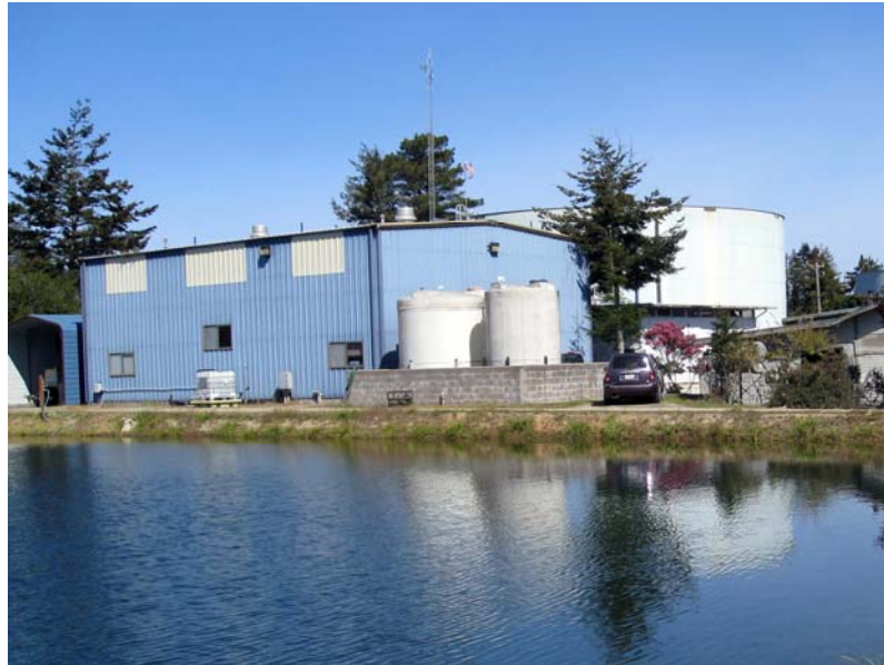
Raw Water Pond
