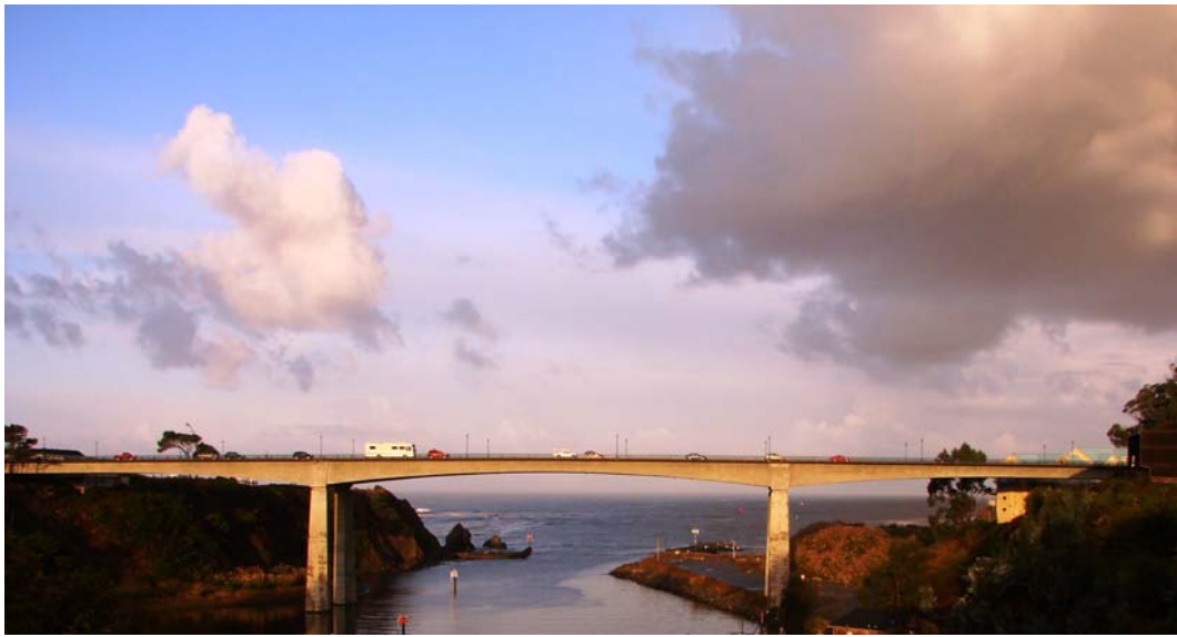
Noyo River Bridge
