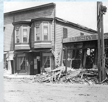
Damage from the Great Earthquake
