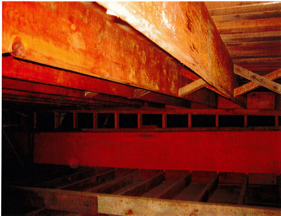
Roof Framing in North Apparatus Room
