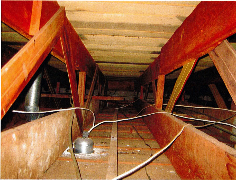
Roof Trusses in Rear Area
