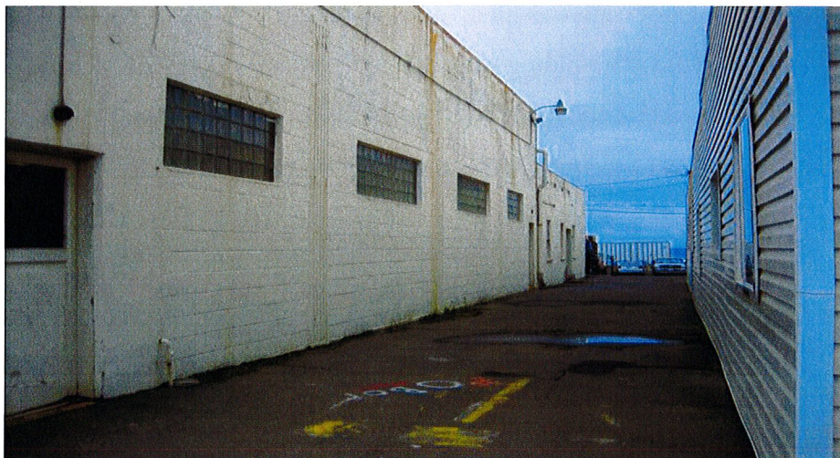
North Wall. Openings in Masonry Wall
