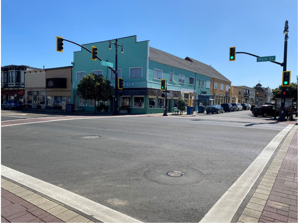
The intersection of Main Street and Laurel Street, looking east
