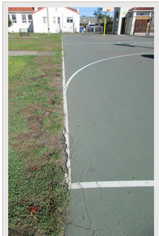
The edge of the existing undersized basketball court
