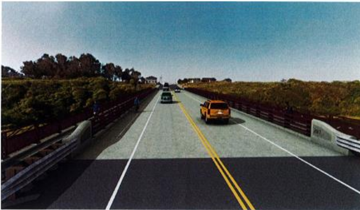
Pudding Creek Bridge: View looking South
