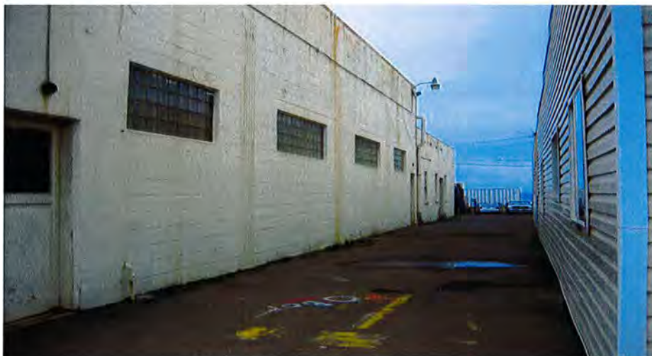
North Wall. Openings in Masonry Wall
