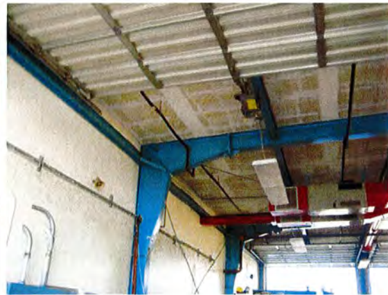
South Wing Interior Frames
