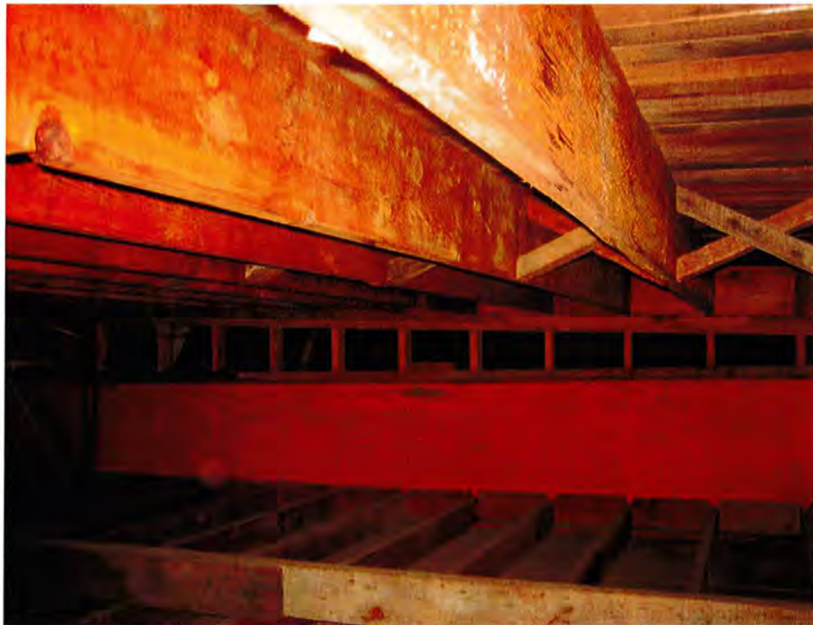
Roof Framing in North Apparatus Room
