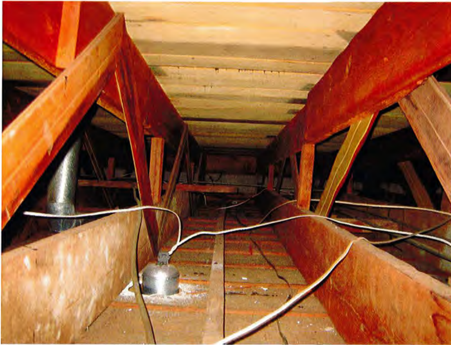
Roof Trusses in Rear Area
