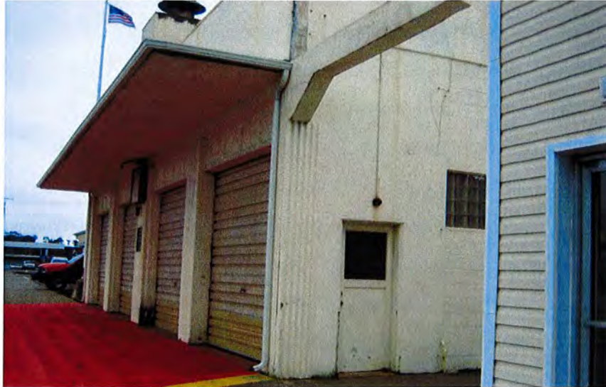
Concrete Frame and Tie Beam on East Wall
