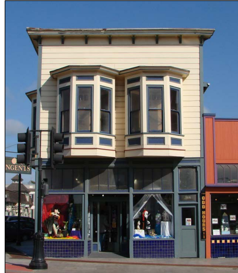
Example of the downtown streetscape
