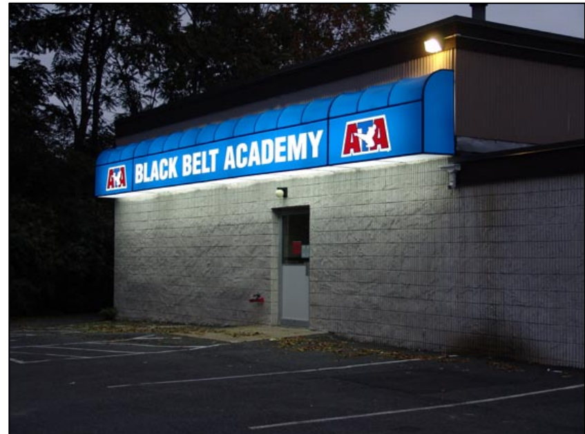
Prohibited awning sign
