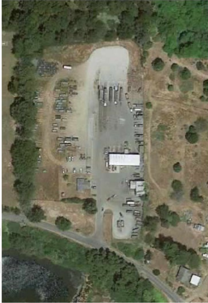
Figure 2. Pudding Creek facility as presented by Diversion Strategies May 2020
