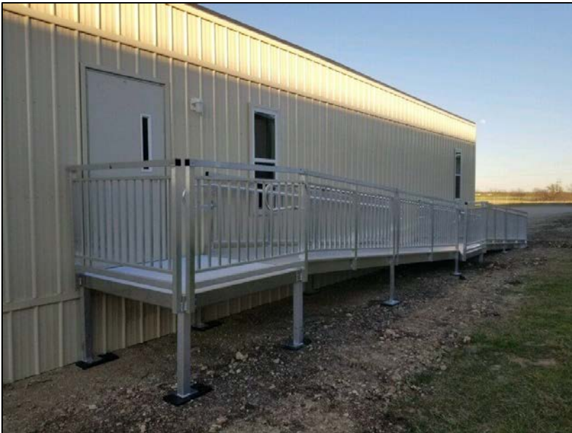
Temporary buildings shall not be visible from public streets
