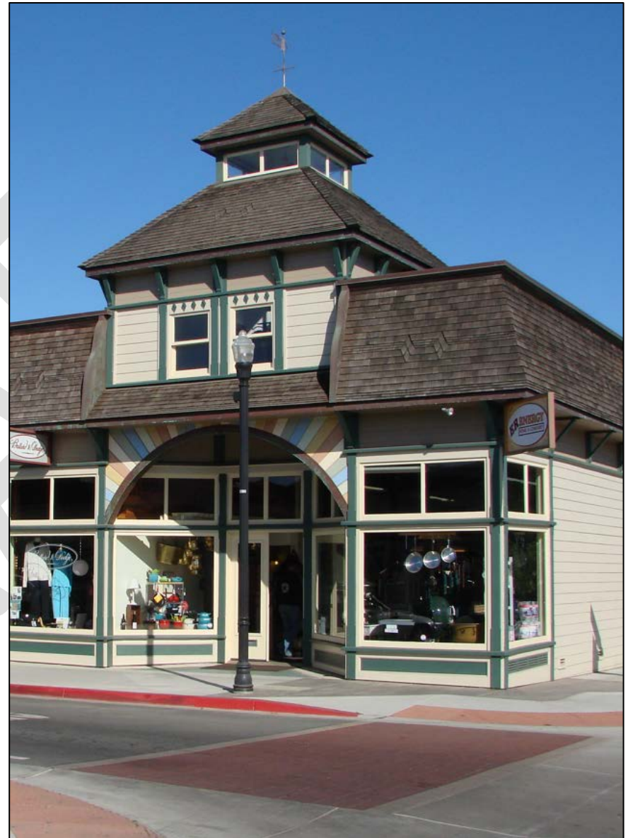
Each storefront should be treated like a small building
