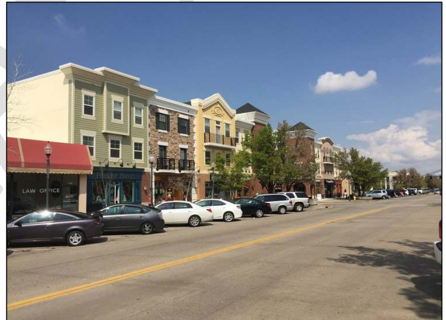
Buildings should be constructed along the front property line(s) with minimal setbacks
