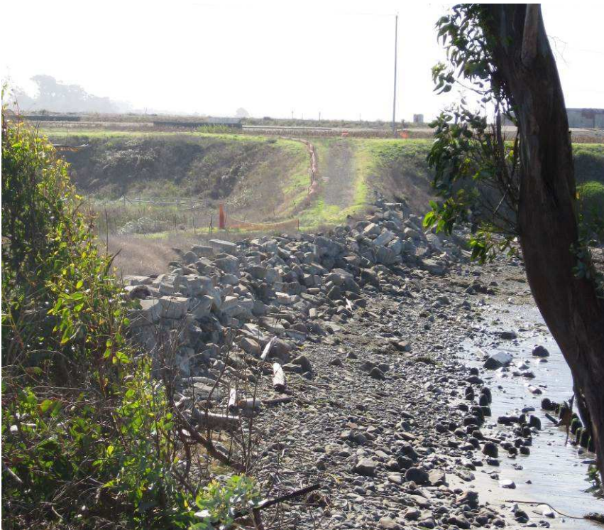
Photograph 3-4 Looking South – Beach Berm, beach and rip rap wall
