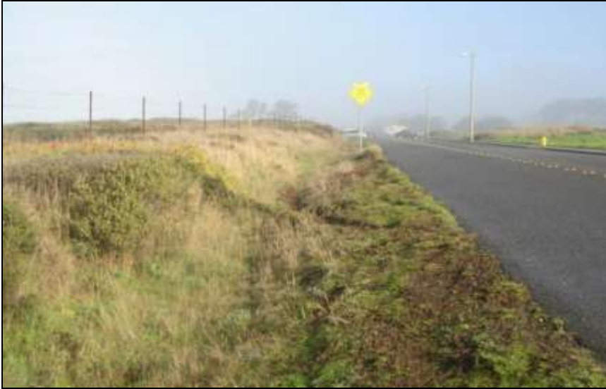
Photograph 3–16. Looking north down the existing drainage ditch parallel to Glass Beach Drive.
