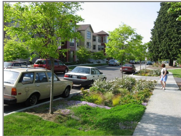
Swales are linear depressions adjacent to the streetscape that can detain and convey stormwater along their length.
