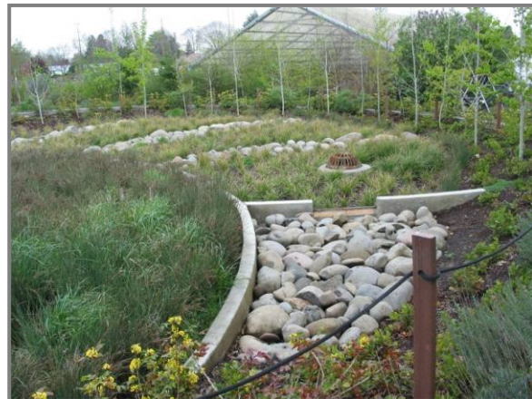
Rain gardens are landscaped planters that are more extensive than storm water planters and typically are designed to infiltrate storm water. They can be located in or adjacent to the street.
