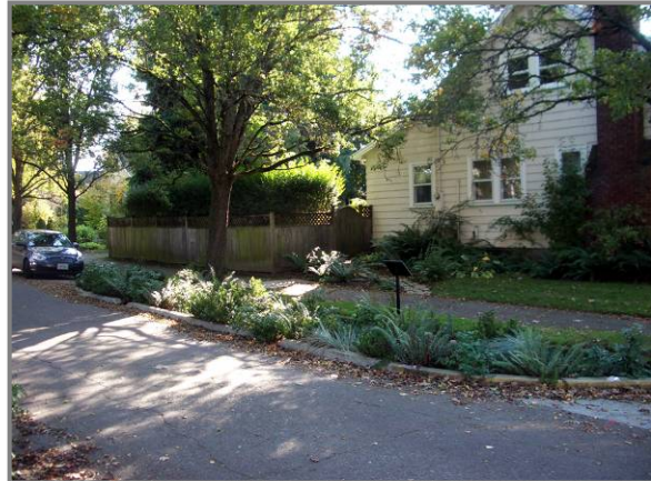
An example of a curb extension with a stormwater planter in Portland, Oregon.
