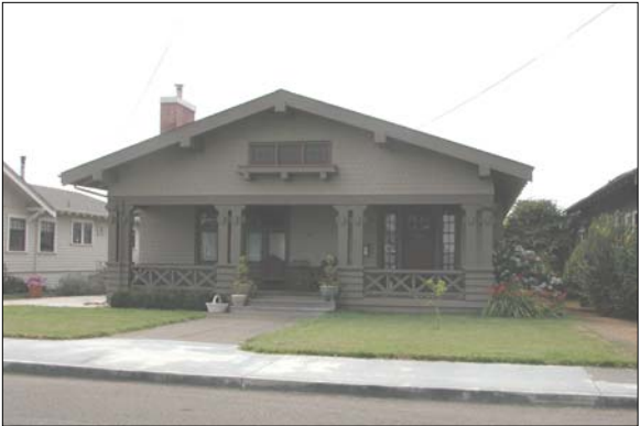
Good example of front porch detail
