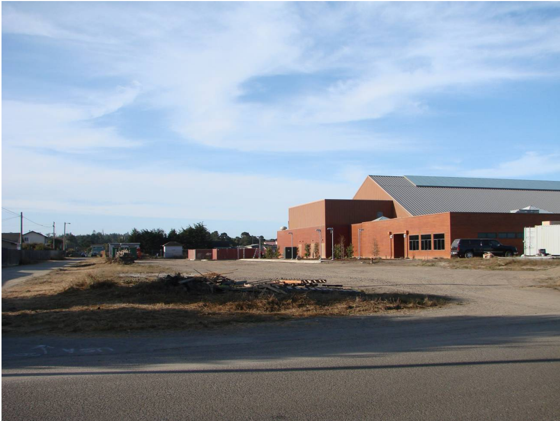
1. View of project area as seen from Willow Street looking south.
