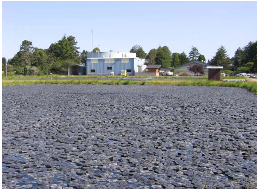
Raw water pond with Hexa Tiles
