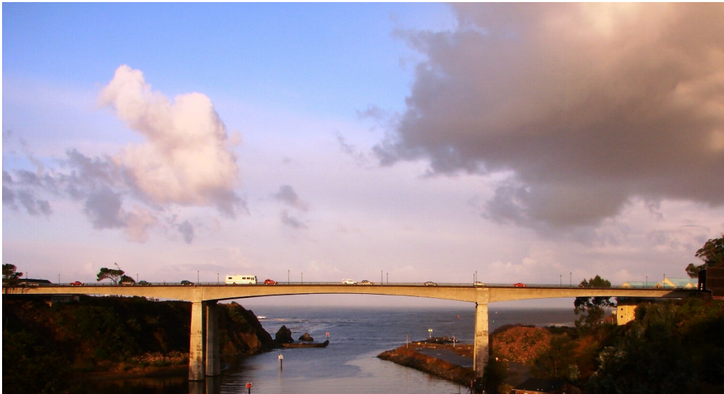
Noyo River Bridge
