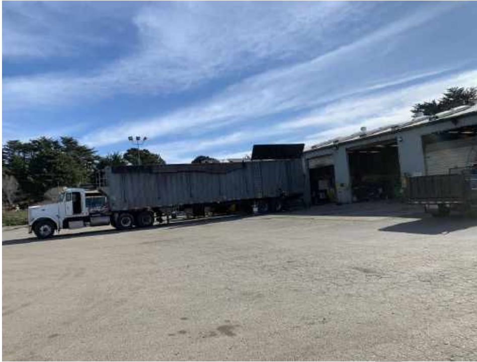
Photo 12: Truck and Maintenance Shop, East Side of Facility
