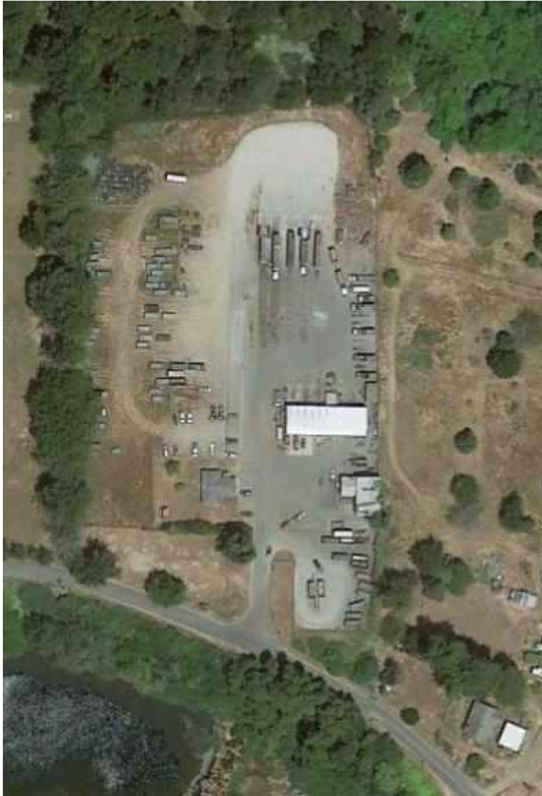
Photo 8: Pudding Creek Facility
