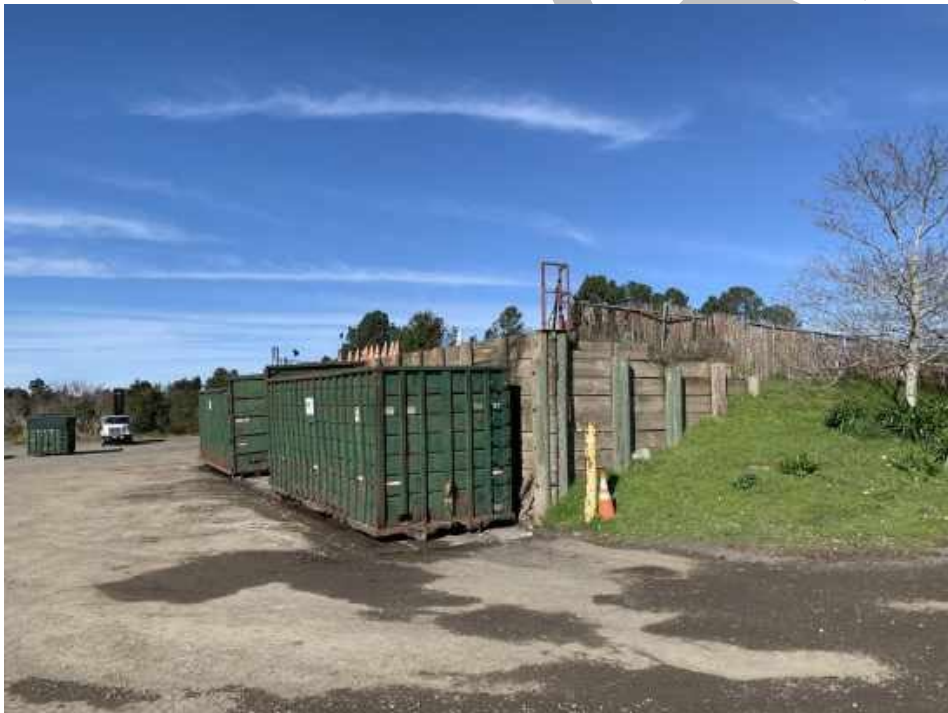
Photo 6: Current Z-wall for Load-out into Debris Boxes
