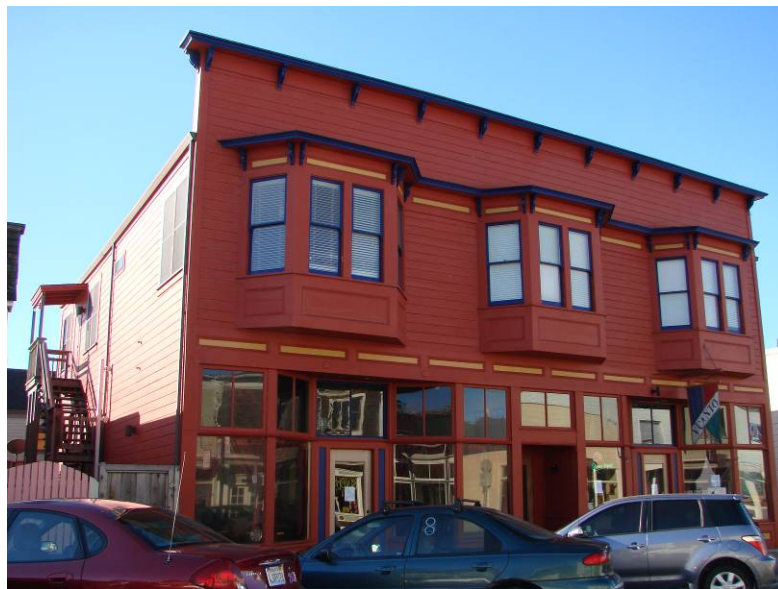
124 Laurel Street: A historically significant structure in the Central Business District
