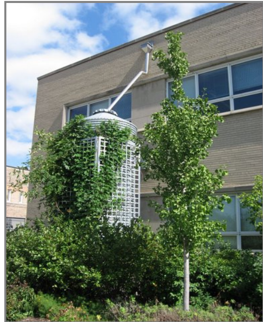
A system that captures rainwater.
